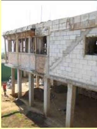
Second Level construction
